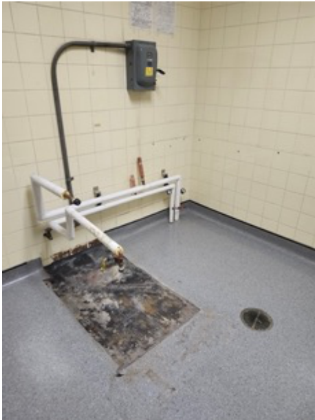
Photograph 1 – View of typical building materials observed within the area and where black floor mastic and beige ceramic tile mastic are asbestos-containing .
