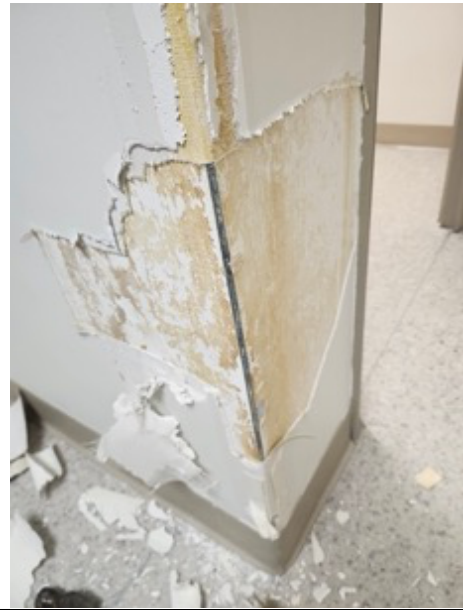
Photograph 6 – View of sampled drywall joint compound and plaster which do not contain asbestos.
